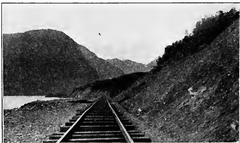
FIG. 376.—The Copper River and Northwestern Railway in the Chugach Mountains of Alaska, where it traverses the stagnant, moraine-veneered, vegetation-covered terminus of Allen Glacier for 5\frac{1}{2} miles. There is ice beneath the rails and ties in the foreground.
